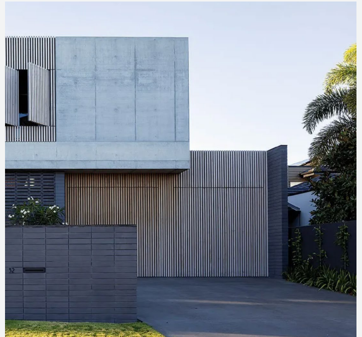
Timber Batten Screen
